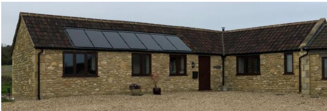
Case officer's site photograph of Bays Corner as built and extended
