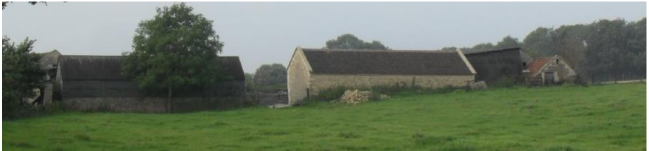
View of north-east elevation of site from existing track from September 2014
